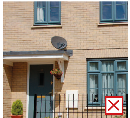
Satellite dishes to be positioned to minimise visual intrusion and away from front elevations wherever possible
