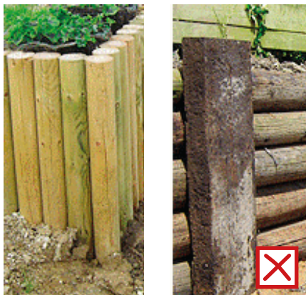
Timber log retaining wall to the public realm will not be acceptable.
