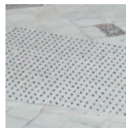
Conservation tactile paving
