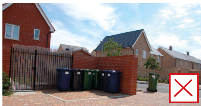
Open bins at main entrance of dwellings / apartment block are not acceptable.
