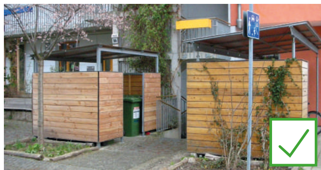
Communal bin stores for apartment blocks must either be integrated with the building and / or designed as a roofed enclosure and sited unobtrusively.
